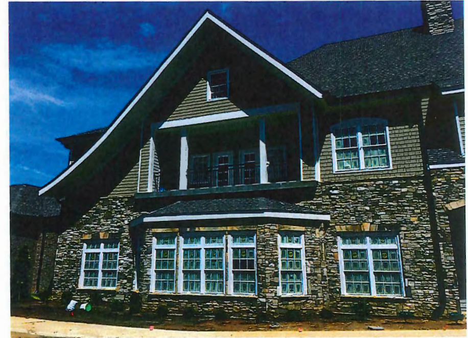
South Elevation at Dining Room Window
