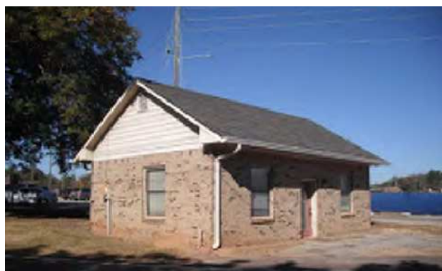
STUCTURE - ON PROPERTY AT NORTHEAST CORNER
