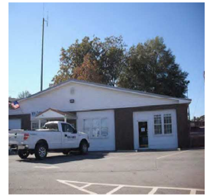
STRUCTURE TO BE REMOVED
