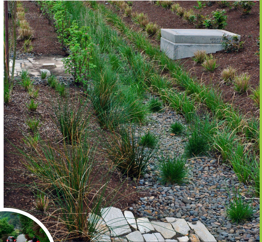
Bioretention cells and rain garden
