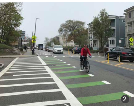
1) Standard continental crosswalk 2) Standard crosswalk with separate bicycle crossing and green conflict point 3) Enhanced crosswalk with brick pavers
