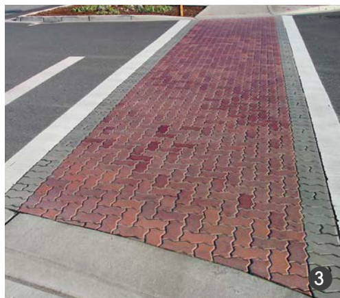
1) Standard continental crosswalk 2) Standard crosswalk with separate bicycle crossing and green conflict point 3) Enhanced crosswalk with brick pavers
