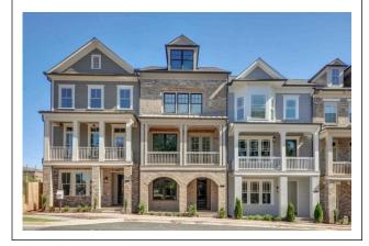
The vertical plane of each dwelling unit's primary front and rear façade shall modulate back and forth a minimum of 2 ft. from the vertical plane of the dwelling unit(s) to either side.
