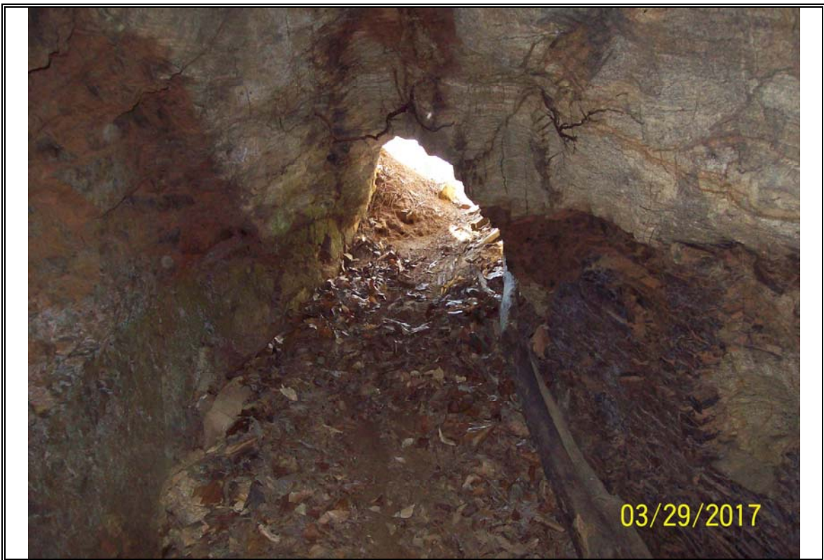
Photo # 4: View from inside mine. Note gray saprolite over most of mine entrance.
