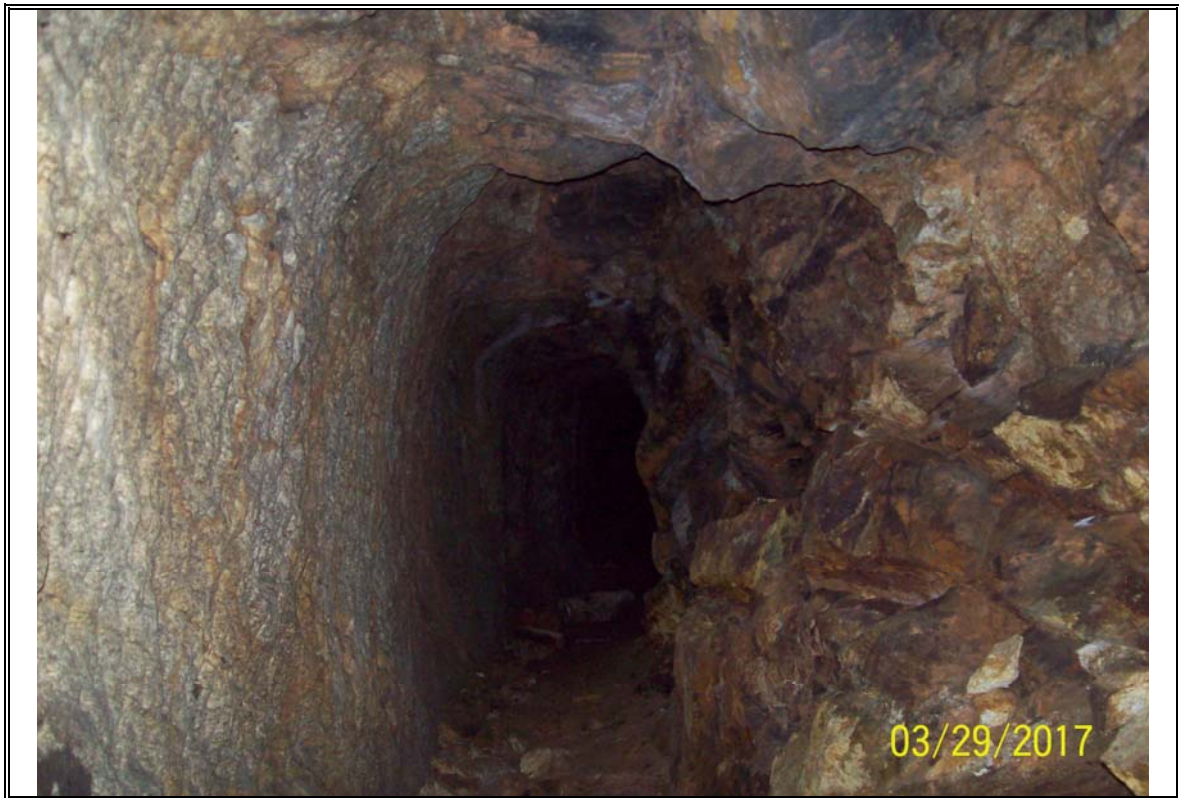
Photo # 5: View of tunnel with gray saprolite to left and highly fractured mica schist and quartzite overhead and right.
