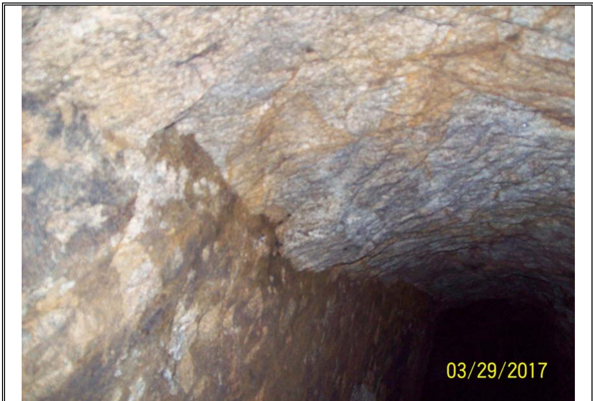
Photo # 6: View of section of tunnel with gray saprolite overhead terminating into plane of mica schist on sidewall.
