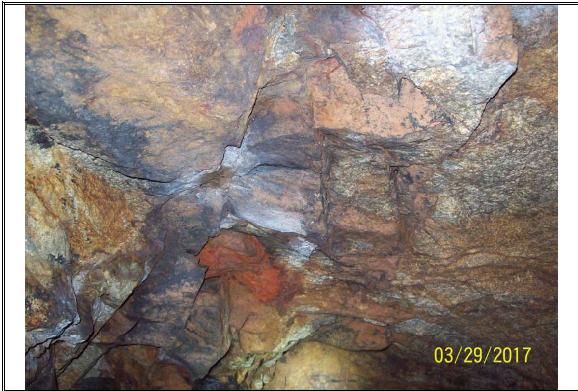
Photo # 9: View of highly fractured mica schist and quartzite in mine tunnel ceiling.
