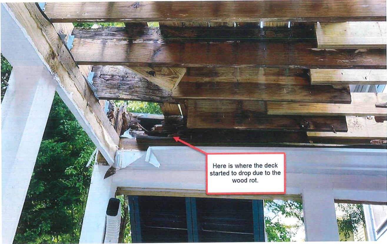
Here is where the deck started to drop due to the wood rot.
