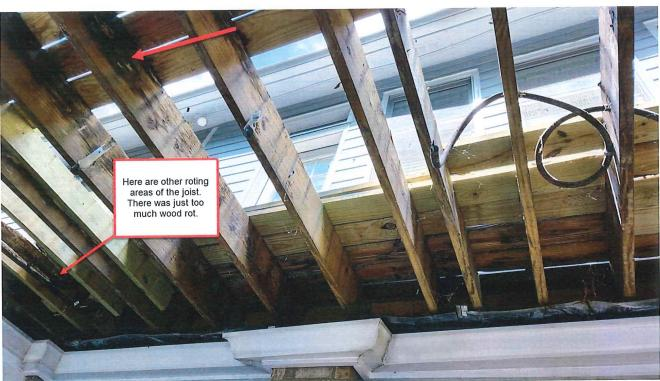
We did not want to run the risk with under decking again, so we thought the best option was to rebuild the deck and add a roof to prevent water from going into the screen porch. The new deck was extended 7 ft to match the existing brick porch underneath. We were unaware that a new permit would be required.
