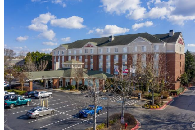
11695 Medlock Bridge Rd Hilton Garden Inn Atlanta North/Johns Creek
