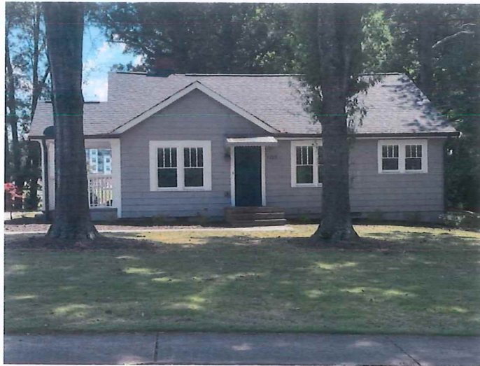
Front View From Sidewalk
