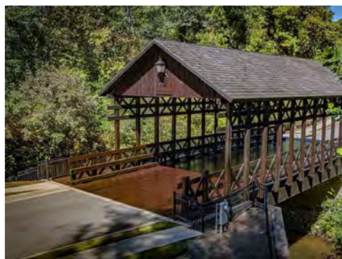
COVERED BRIDGE AT ENTRY CREEK CROSSING
