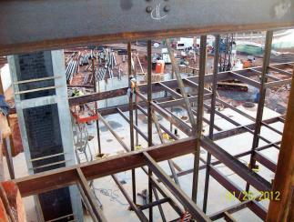
Despite the wet winter, the steel framing is progressing rapidly. In the photos, the steel floor joists are welded in place that will create the two floors as seen from West Broad St. In the second photo we are looking down from the top of the roof and in the distant upper right corner we can see the amphitheater and the amenity detention pond which is nearly complete.
